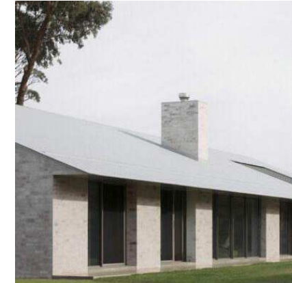
PC01 / RS01 ROOF SHEETING AND MATCHING TRIMS (INCLUDING GUTTERS, DOWNPIPES, AND FLASHINGS) COLOUR TBC (TO MATCH WALLS)
