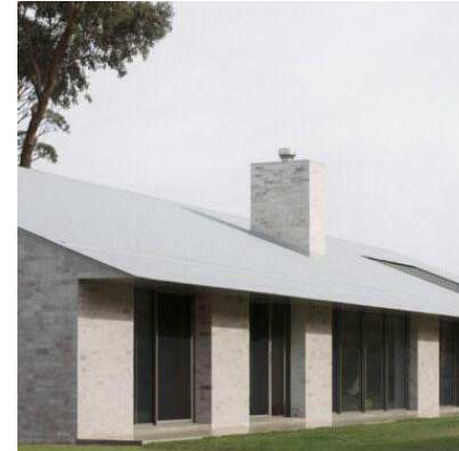
PC01 / RS01 ROOF SHEETING AND MATCHING TRIMS (INCLUDING GUTTERS, DOWNPIPES, AND FLASHINGS) COLOUR TBC (TO MATCH WALLS)
