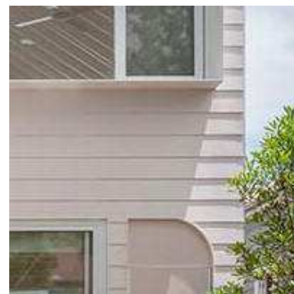
CL01 LIGHTWEIGHT HORIZONTAL WEATHERBOARD CLADDING SELECTION & COLOUR TBC
