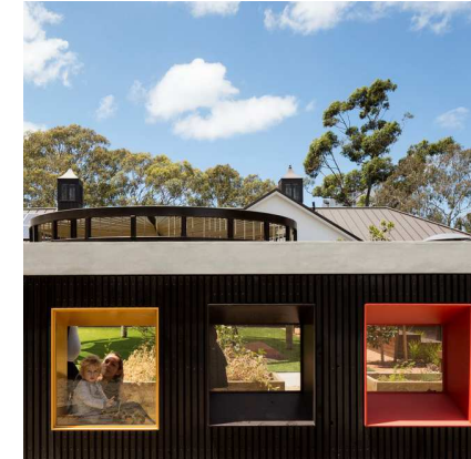
PC02 FOLDED ALUMINIUM WINDOW HOODS (POWDERCOAT FINISH) VARIOUS COLOURS
